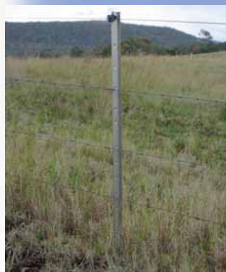
This four strand fence (1 plain 2 barb 1 plain) where the top wire can be electrified for extra security if needed has proven sufficient to control cattle and is a much safer option for wildlife.
