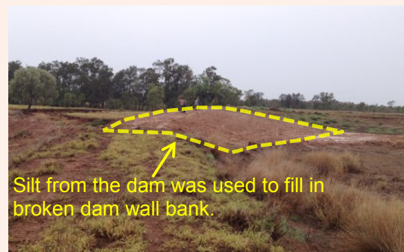
Figure 3: After photo of dam bank reinstatement
