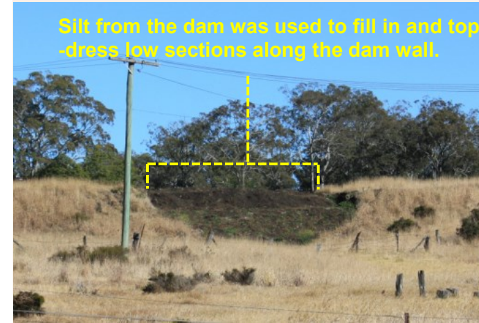
Figure 4: Reinstated low section of dam
